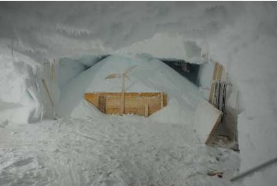
The EGRIP drill site after casing extension and backfilling with snow, July 2024.
